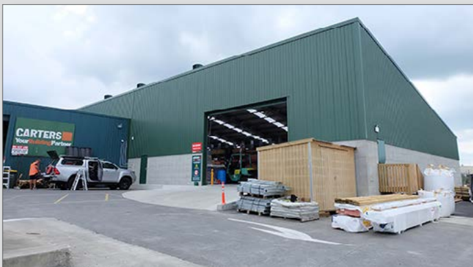
Clearspan monopitch at 21m wide x 32m long, high stud, drive-thru commercial warehouse for Carters Pukekohe, Auckland.
