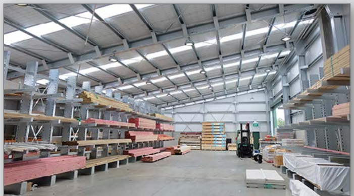
Clearspan monopitch at 21m wide x 32m long, high stud, drive-thru commercial warehouse for Carters Pukekohe, Auckland.
