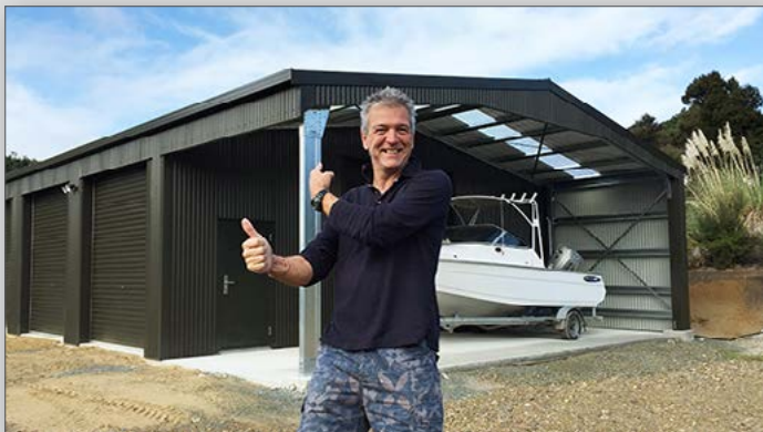
10m wide x 18m long x 3.4 high shed incorporating both secure and open bay storage.
