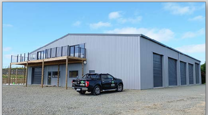
22m wide x 30m long x 5.5 high workshop with mezzanine office floor.
