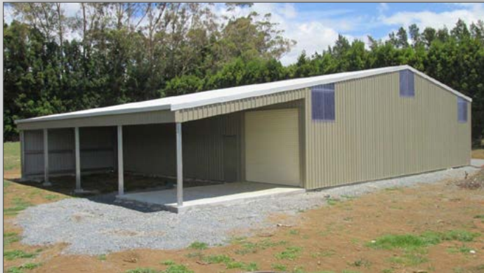
16m x 16m secure workshop with 6m lean-to. Added feature is the clear-lights.
