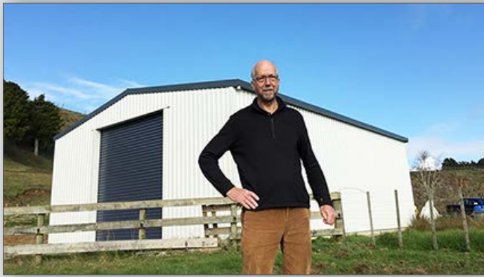
10m wide x 14m long x 4.3m high shed for farm machinery.
