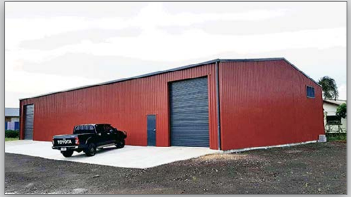
16m wide x 30m long x 4.3 high warehouse in Samoa.
