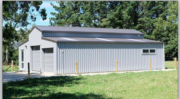
9m wide x 12m long x 3.6 high Heritage Barn.
